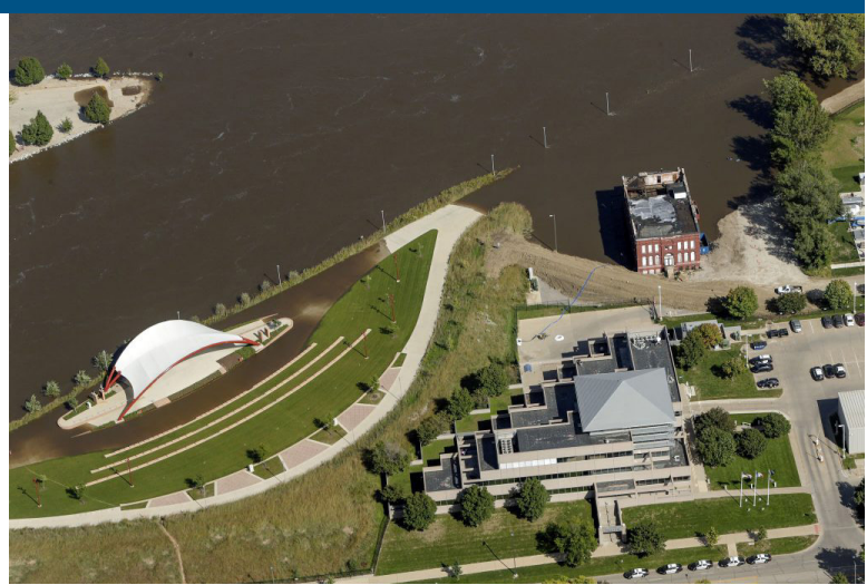
The McGrath Amphitheatre (left) takes on water as does the Knutson Building (upper, right) in an aerial photograph on Monday, Sept. 26, 2016. Cedar Rapids Police Department is at lower, right. (Jim Slosiarek/The Gazette)
