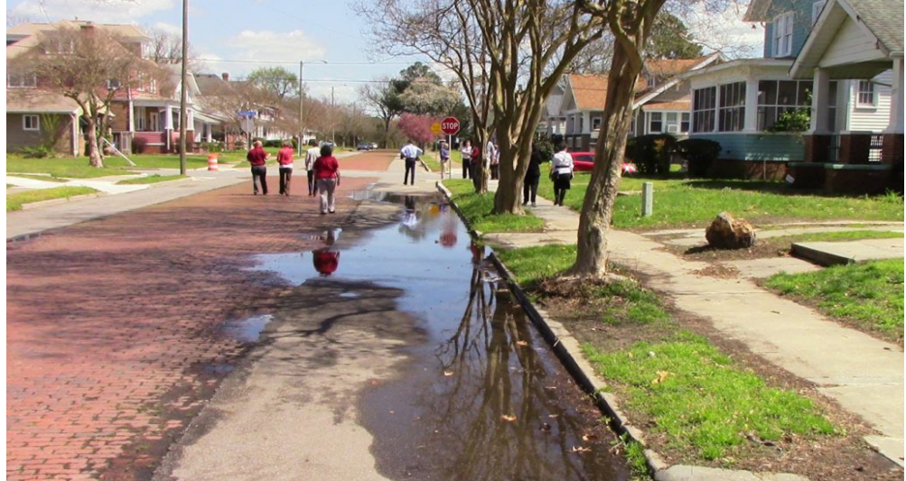
Overflowing stormwater system in Chesterfield Heights. Credit: EPA
