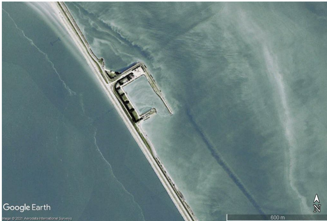
Houtrib Dike before reinforcement. Source: Google Earth.
