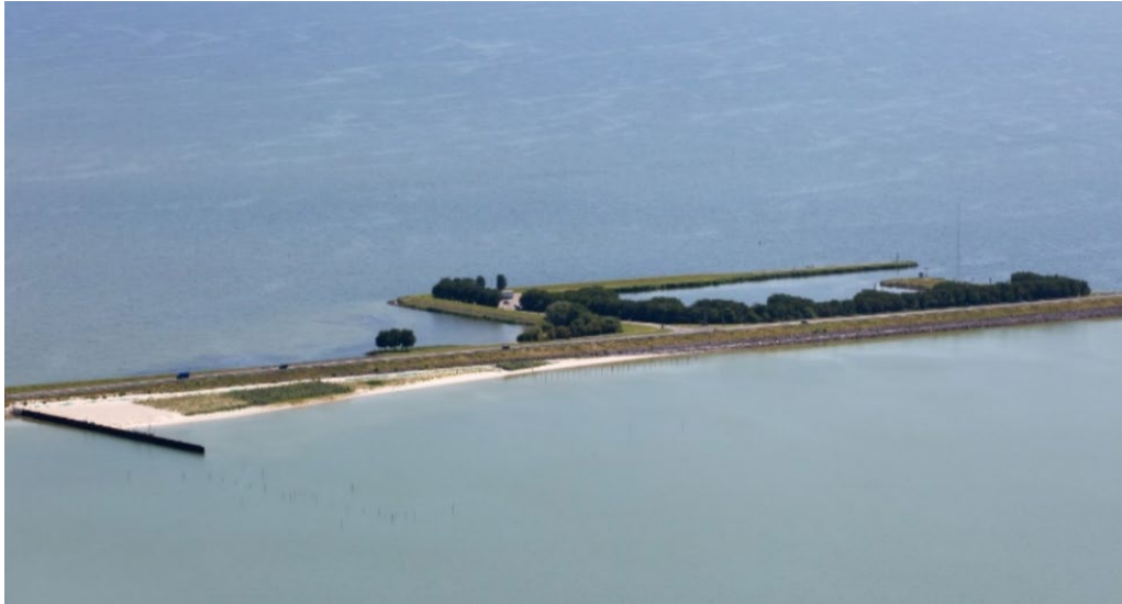
Houtrib Dike trial section in 2017. Source:
