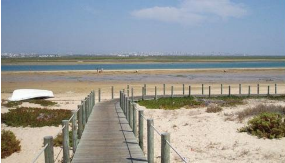
Praia do Faro after the implementation of the elevated wooden pathway. Source: https://www.coastal-management.eu/measure/example-cost-effectiveness-analysis-wooden-path-over-dune-praia-de-faro-pt
