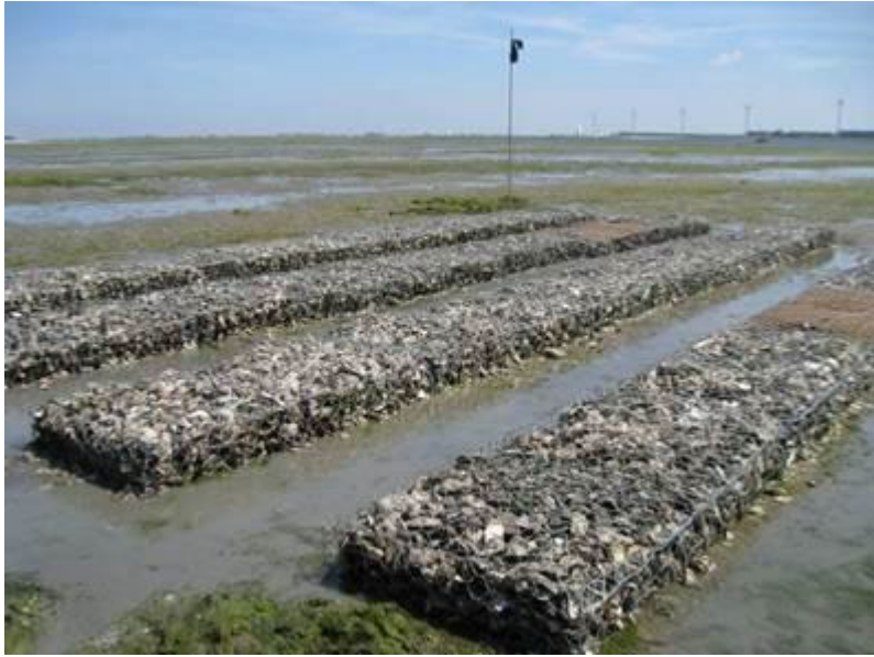
Small-scale pilot on a salt marsh area. Source: https://www.ecoshape.org/en/cases/shellfish-reefs-as-shoreline-protection-eastern-scheldt-nl/construction-phase/
